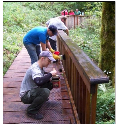
Sam Packham crew staining puncheon.
