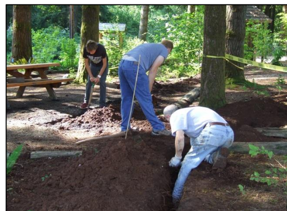
Installation of the irrigation system.
