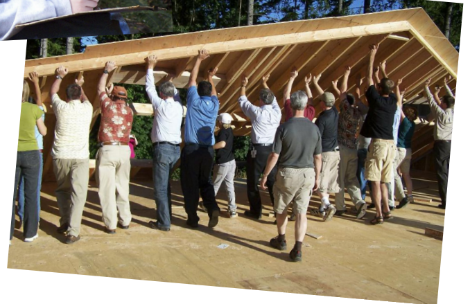
Raising one of the walls at the new education building
