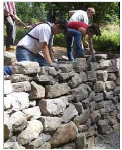
The Clackamas County Youth Corps crew was given 35 tons of rock and a simple picture of how to stack a dry wall, and built the wall like a puzzle—sometimes pulling rock out to fit another into place.
